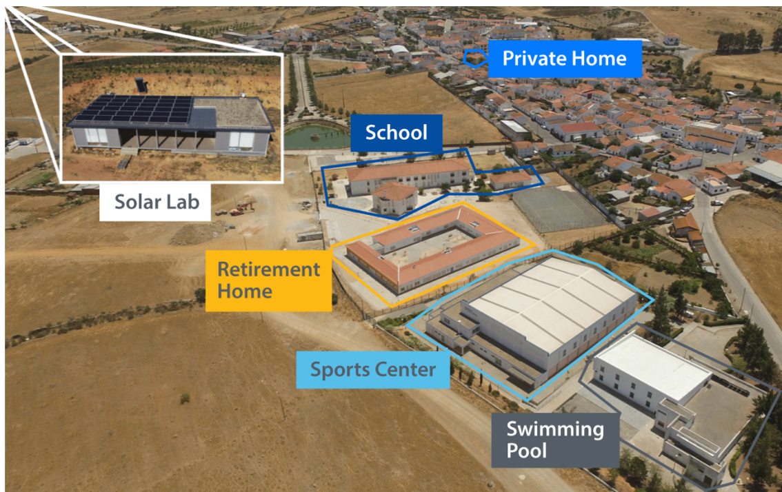
Figure 6 - Overview of buildings included in the Pilot Site at Martim Longo
