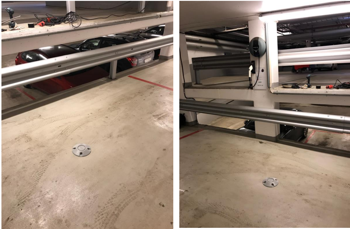
Figure 6: Mounted PNI PlacePod parking sensor at Hoegh Eiendom
