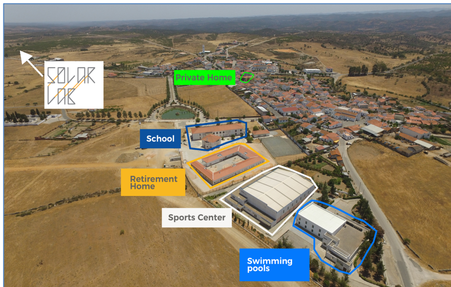
Figure 4-1 Pilot Site Overview
