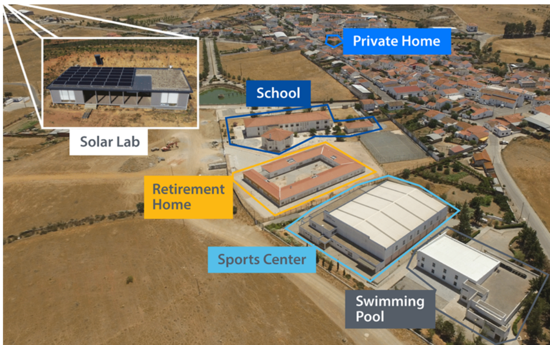
Figure 4: Overview of buildings included in the Pilot Site at Martim Longo
